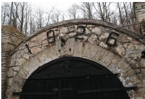
Fig. 2 Access to the mine (the photo taken by the authors)
